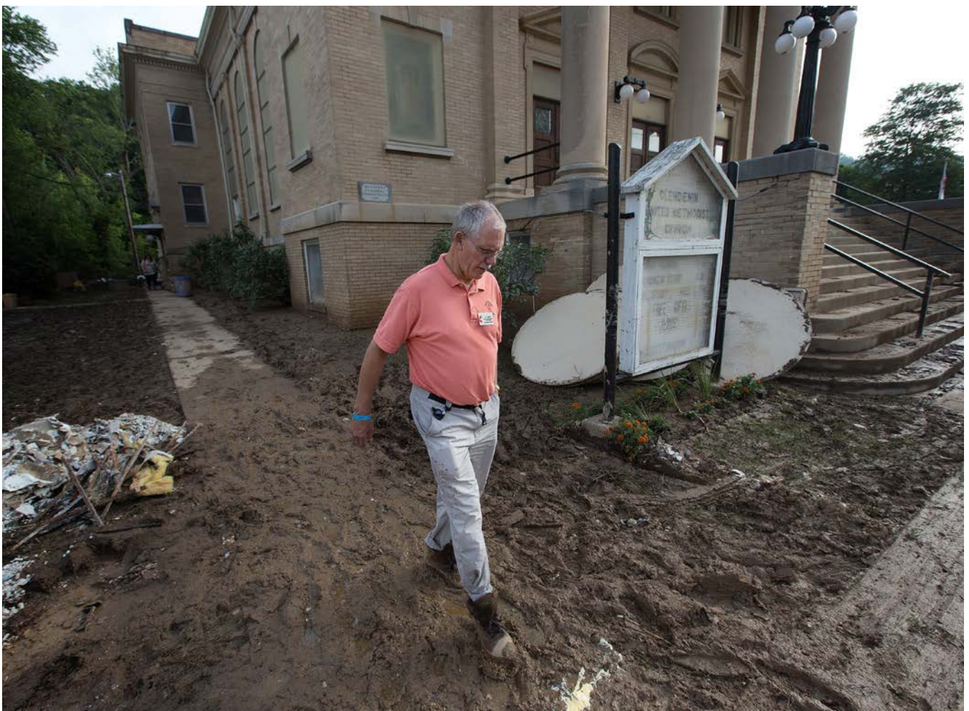
The Rev. J.F. Lacaria surveys flood damage at Clendenin (W. Va.) United Methodist Church. Photo by Mike DuBose, UMNS.
